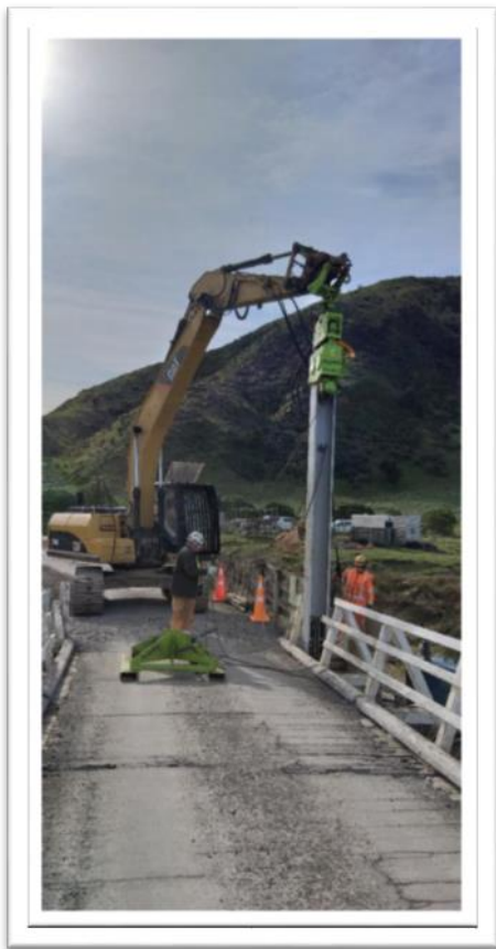
Pile driving Tora farm Settlement bridge.
